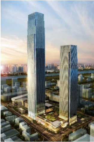
Exterior, Niccolo Changsha
